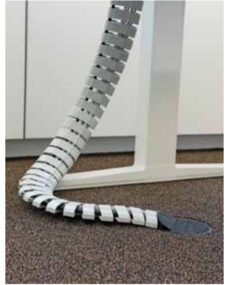
EVoline floor outlet with EVoline WireLane placed according to layout plan.
