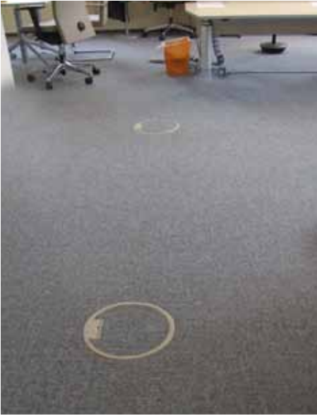
At the time of moving into a representative new office building. Sub-floor boxes are installed in a grid pattern.
