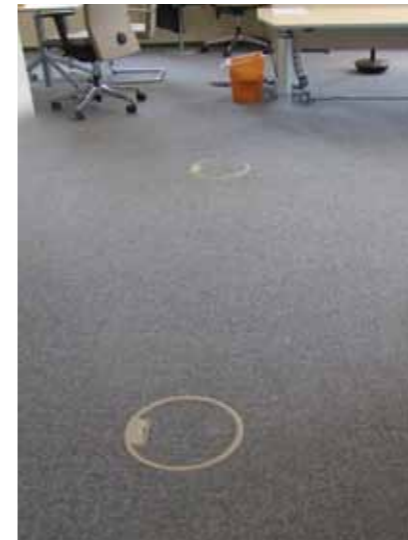
Moving into a prestigious new office building – floor boxes installed in a grid pattern
