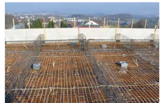
Concrete core activation in the ceiling before application of concrete.
